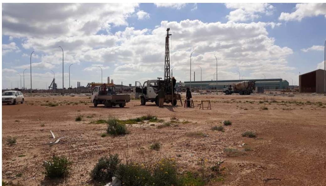
Photo No. 6: Borehole#06 (Misurata free zone, Misurata city). Date:06/03/22
