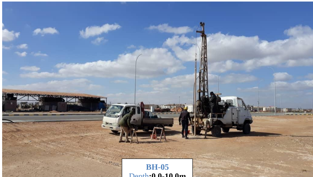
Figure 4: The boring test is being performed on the site (Misurata free zone area).
